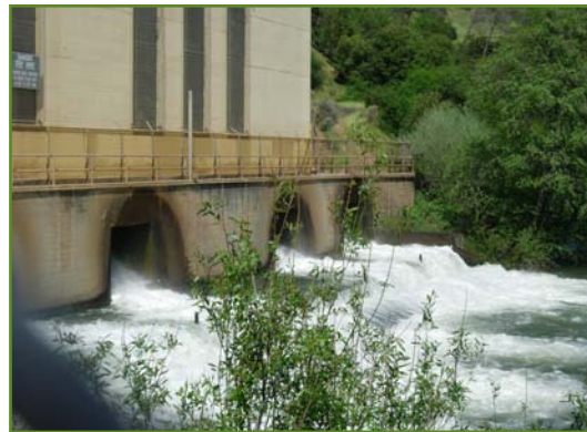
PG&E Electra Powerhouse
